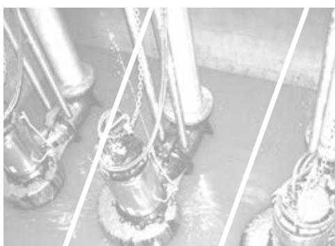
Wastewater Transport and Treatment
